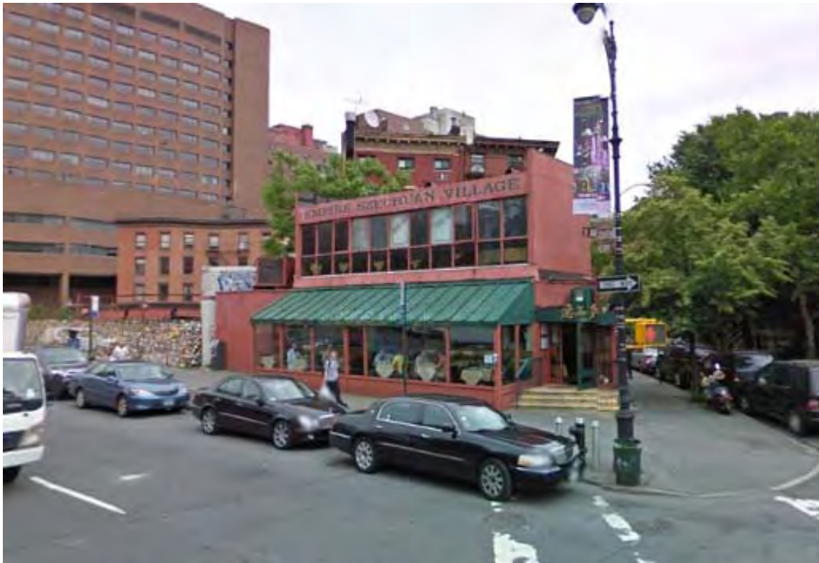
173 Seventh Avenue South today (source: Google Maps)
