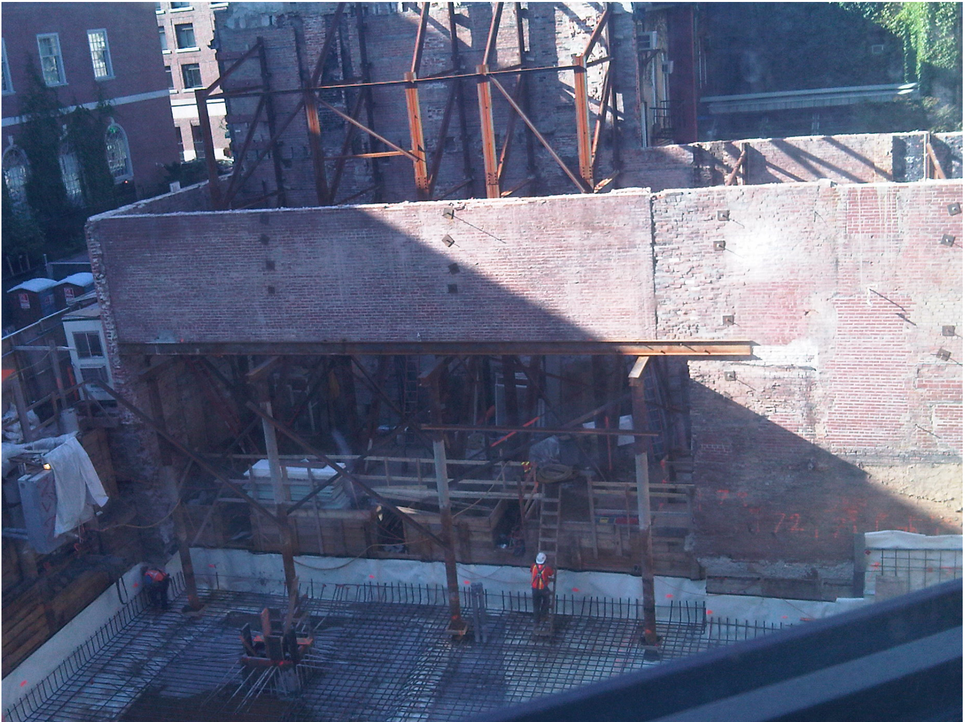
Demolition of Provincetown Playhouse & Apartments - 09/01/2009
